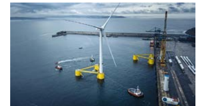
Floating foundation system for offshore wind power plants (Photo courtesy of Principle Power. Artist: DOCK90)
