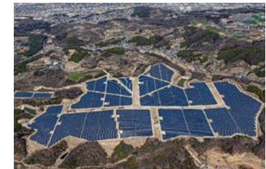
Annaka Solar Power Plant, one of the largest-capacity PV plants in the Kanto Region
