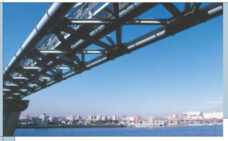
December 1999 saw the completion of the Keihin and Yokohama transmission pipelines. Tokyo Gas now boasts a 300km-long supply loop encircling the greater Tokyo area. Pictured is the Tsurumi River Bridge, which was built for the Keihin Transmission Pipeline.
