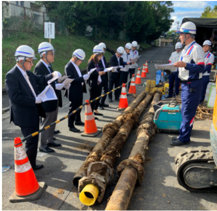
Replacement work on aged gas pipelines during a site visit (Tokyo Gas Network)
