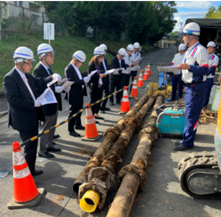
Replacement work on aged gas pipelines during a site visit (Tokyo Gas Network)
