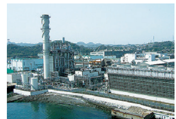
Tokyo Gas Yokosuka Power Co., Ltd.
