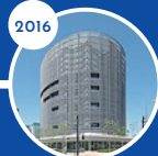
Toyosu Smart Energy Center
