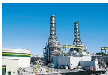
Kawasaki Natural Gas Power Generation Co., Ltd.
