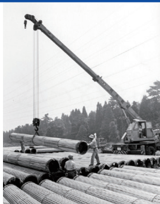
Chiba main pipeline work
