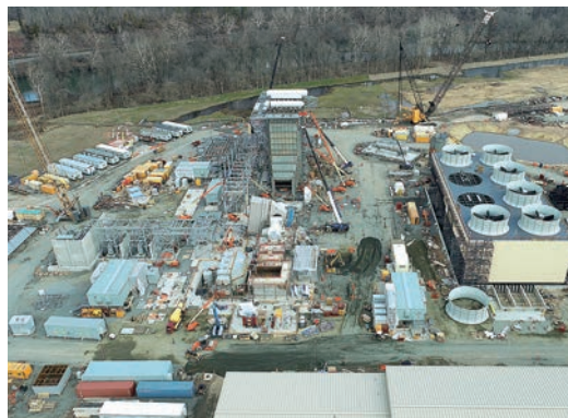
Birdsboro Power Plant (under construction)
