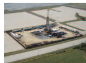
Shale gas development project in the Barnett Basin
