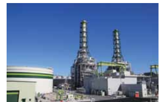
4 Kawasaki Natural Gas Power Generation Co., Ltd.
