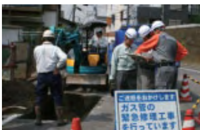
Emergency Repair Work on Gas Pipes
