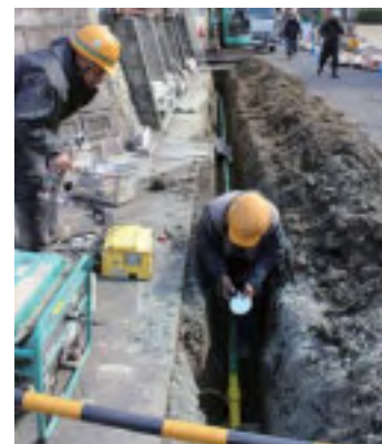
Pipeline Restoration Work
