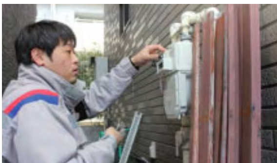
Restoration Work at a Customer's Home
