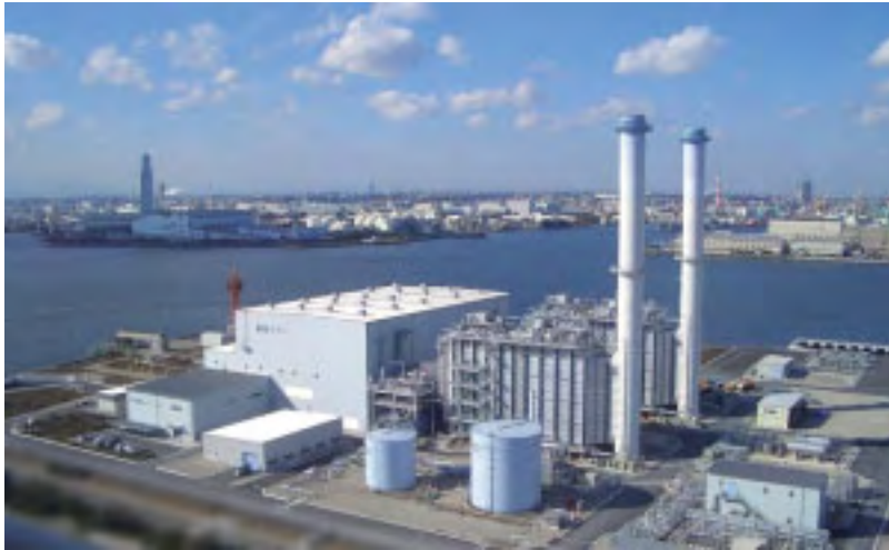
No.1 and No.2 units at the Ohgishima Power Station (Each has an output capacity of 407.1 MW)
