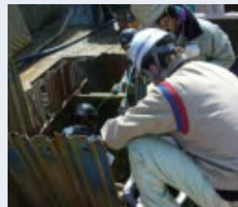
Repairing a Low-pressure Supply Pipe
