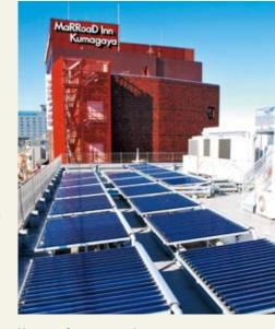
Heat transfer system at the Company's Kumagaya Branch. Solar heat from a solar heat collector (front) installed on the roof of the Company's Kumagaya Branch is transmitted to a nearby hotel (back) through heat transmission lines. This is the first system in Japan that transmits solar heat among private-sector buildings with different owners.
