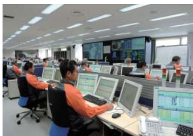
Safety control center
