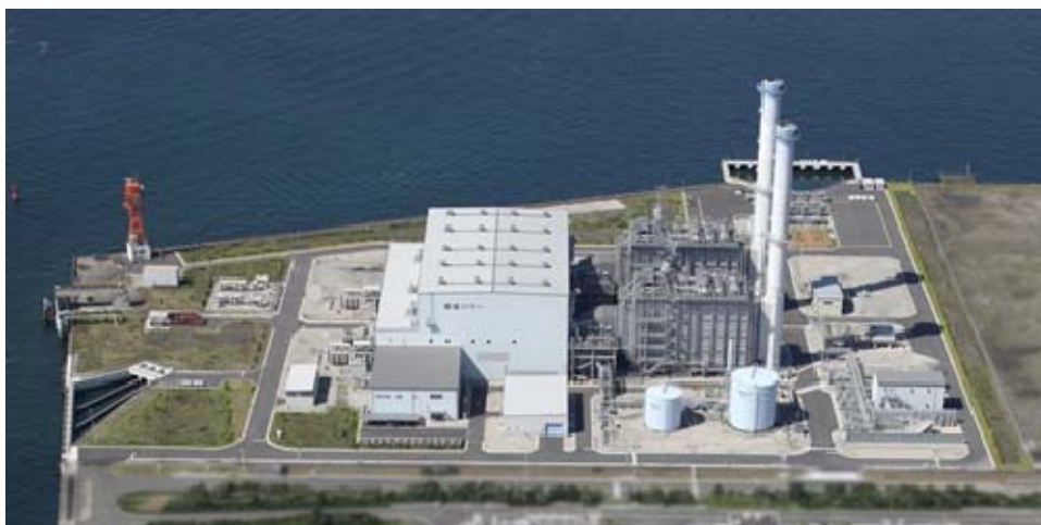
Ohgishima Power Station at present (Front; Unit 1, Back; Unit 2)
