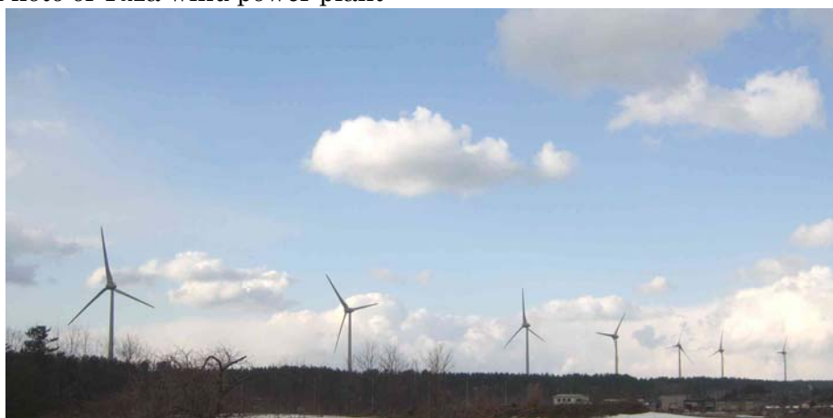
Photo of Yuza wind power plant
