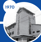
1970 Kuramae Kokugikan First gas heating and cooling system
