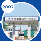
Hydrogen filling station
