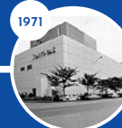
1971 The old Shinjuku District Heating and Cooling Center
