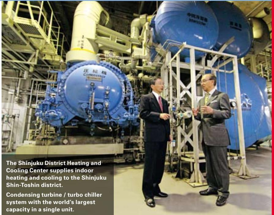
The Shinjuku District Heating and Cooling Center supplies indoor heating and cooling to the Shinjuku Shin-Toshin district. Condensing turbine / turbo chiller system with the world's largest capacity in a single unit.
