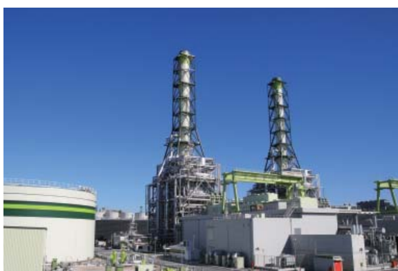
Kawasaki Natural Gas Power Generation
