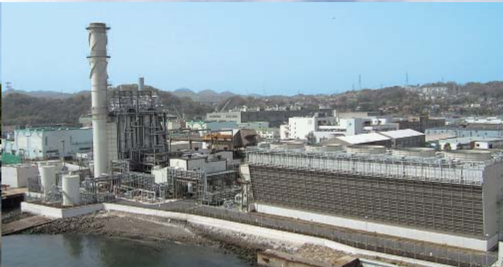
Tokyo Gas Yokosuka Power
