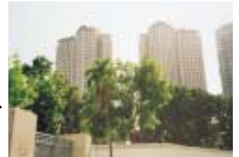
► Feasibility study site for the installation of a centralized district cooling and power supply system in Manila
