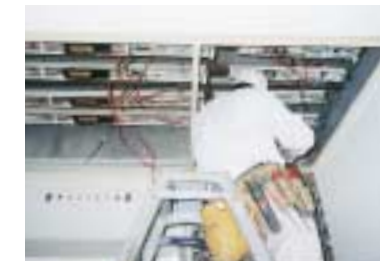
Replacement of a PCB-containing fluorescent lamp ballast
