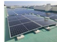
CO 2 -SUICOM blocks supporting solar panels at Motomachi Elementary School in Yokohama
