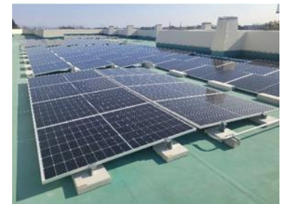
CO 2 -SUICOM blocks supporting solar panels at Motomachi Elementary School in Yokohama
