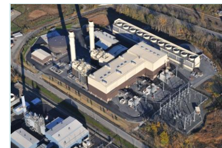
< Empire power plant > (October, 2016)
