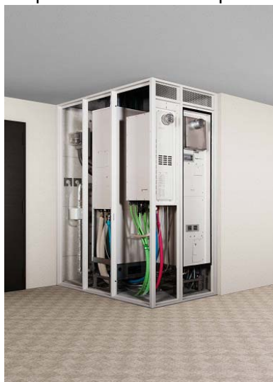
Pipe shaft with doors open
