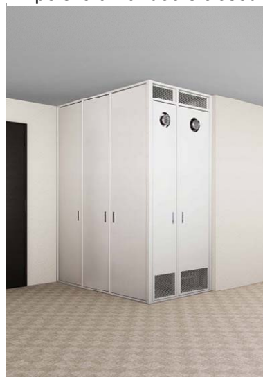
Pipe shaft with doors closed
