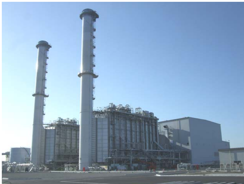
Ohgishima Power Station (Unit 2: front side facility)
