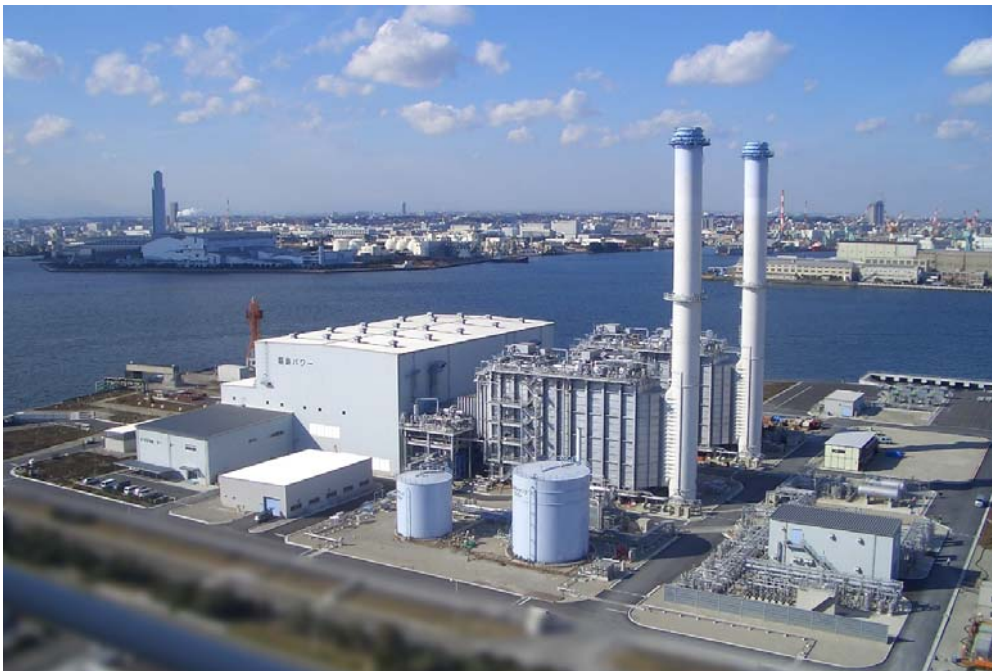
Ohgishima Power Station (Unit 1: front side facility)
