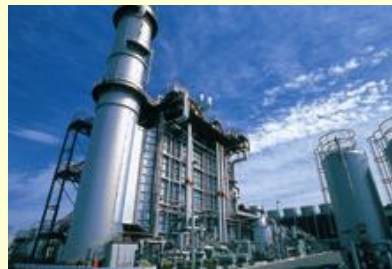
Tokyo Gas Baypower (0.10 mil. kW, 100% stake)
