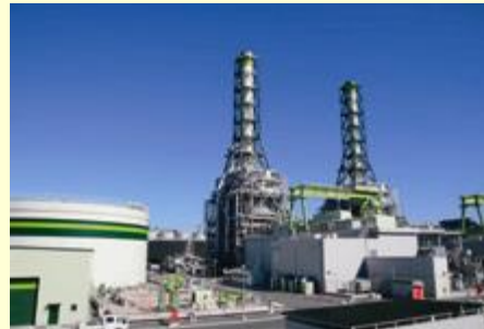
Kawasaki Natural Gas Power Generation (0.80 mil. kW, 49% stake)
