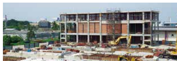
Designed to supply electric power and steam, the energy control center under construction
