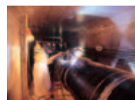
Construction of Keihin Trunk Line
