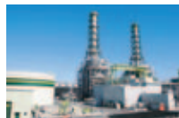
Kawasaki Natural Gas Power Generation Co., Ltd.
