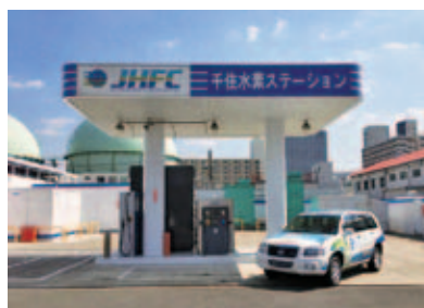
Hydrogen refueling station
