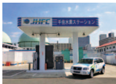
Hydrogen refueling station
