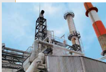
Boiler No. 2, which was successfully lit using natural gas
