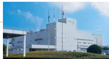
Kao's Kashima Plant
