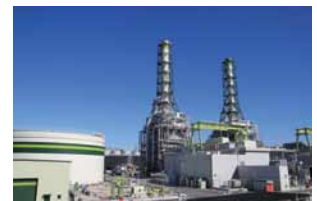
4 Kawasaki Natural Gas Power Generation Co., Ltd.
