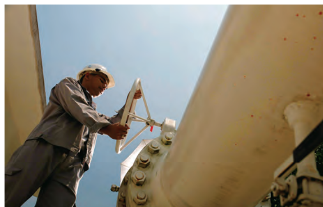
Gas Malaysia Bhd. employee operating a pipeline valve
