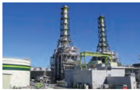
Kawasaki Natural Gas Power Generation Co., Ltd.
