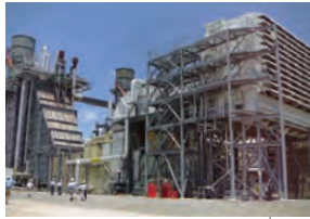
Mexico Bajio Natural gas power generation (Tokyo Gas interest: 49%)
