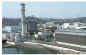
Tokyo Gas Yokosuka Power Co., Ltd.
