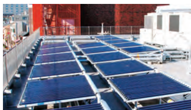
Solar heat collector
