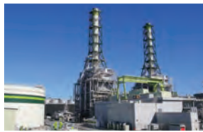
Kawasaki Natural Gas Power Generation Co., Ltd.
