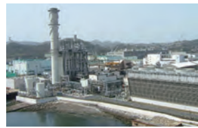
Tokyo Gas Yokosuka Power Co., Ltd.
