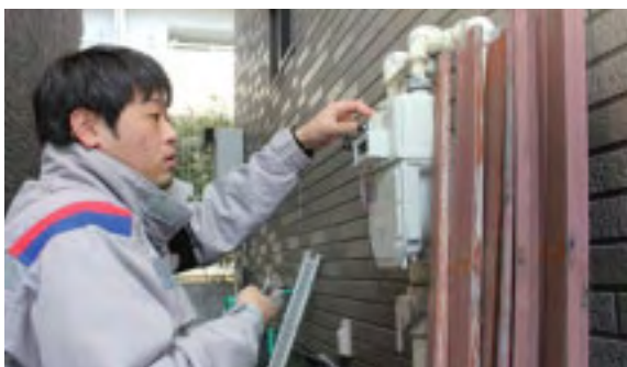
Restoration Work at a Customer's Home
