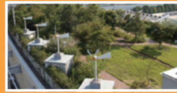
Biotope on the roof of the Energy & Earth Exploratorium
