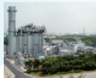
Power plant of Tokyo Gas Bay Power Co., Ltd.
