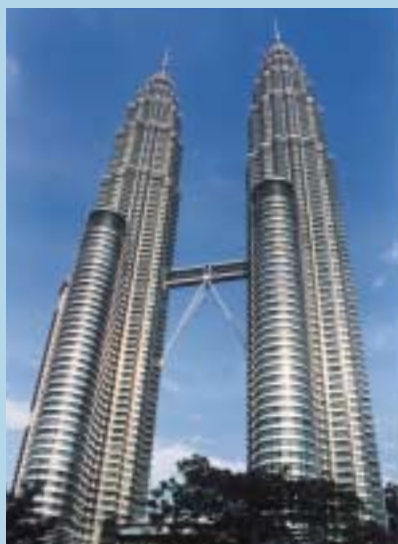
The Petronas Twin Towers, the tallest buildings in the world, are supplied with chilled water by a gas district cooling (GDC) system.
