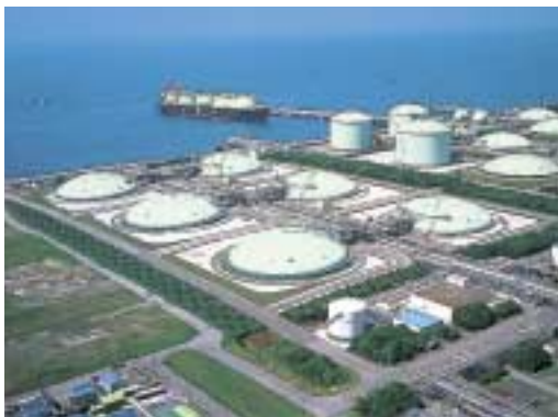
The Sodegaura LNG Terminal is the world's largest LNG receiving terminal.
